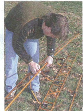
Figure 4 Adding the other I-beam
